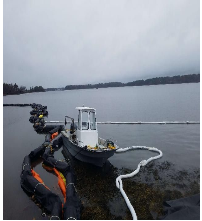
Fig 18: Crew installed second boom around perimeter of site. Viewing north. (11-20-19).
