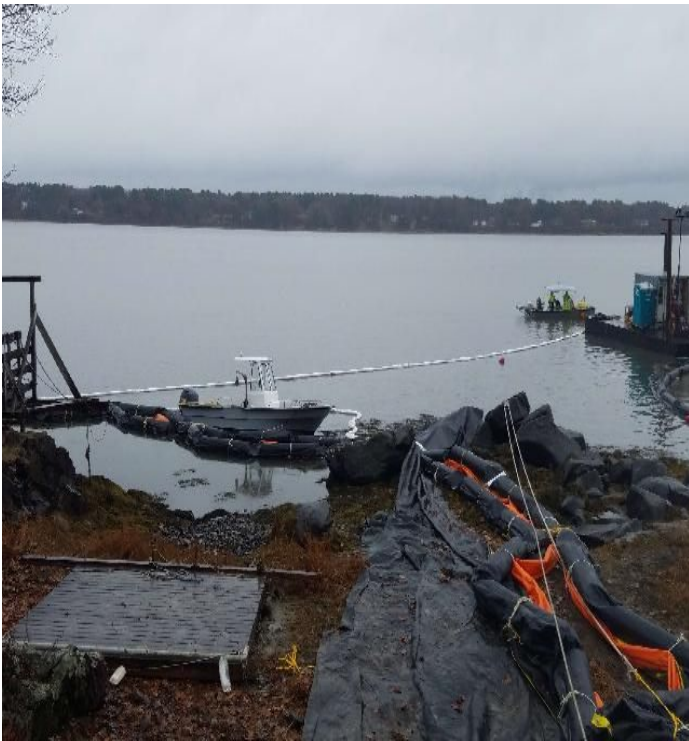
Fig 19: Crew installed second boom around perimeter of site. Viewing east. (11-20-19).
