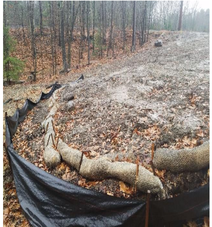
Fig 10: Sediment controls installed downslope of Str. 29. Mulch/straw is recommended. Viewing southeast. (11-19-19).
