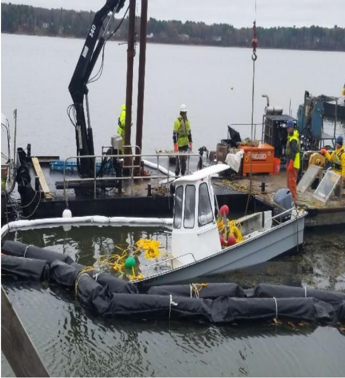
Fig 17: Dewatering capsized boat. Viewing east. (11-20-19).
