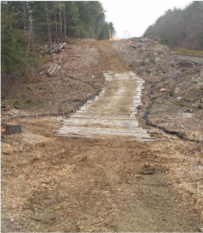
Fig 7: Matted access road through wetland DW91. Viewing north. (11-18-19).
