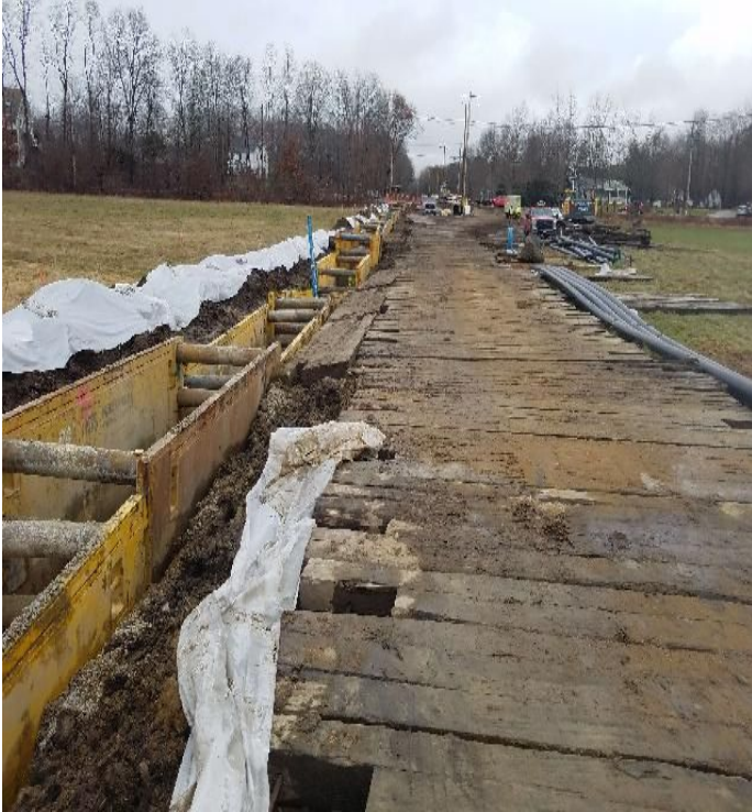
Fig 13: Trenching at Frink farm. Viewing east. (11-19-19).
