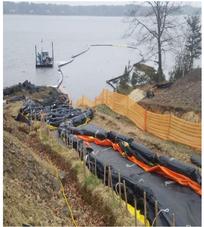
Fig 8: Mackworth assembling turbidity curtain at Getchell property/west side of the Bay. (11-18-19).
